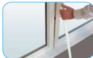
Once locked into position the buttons are used to locate the cover strip
